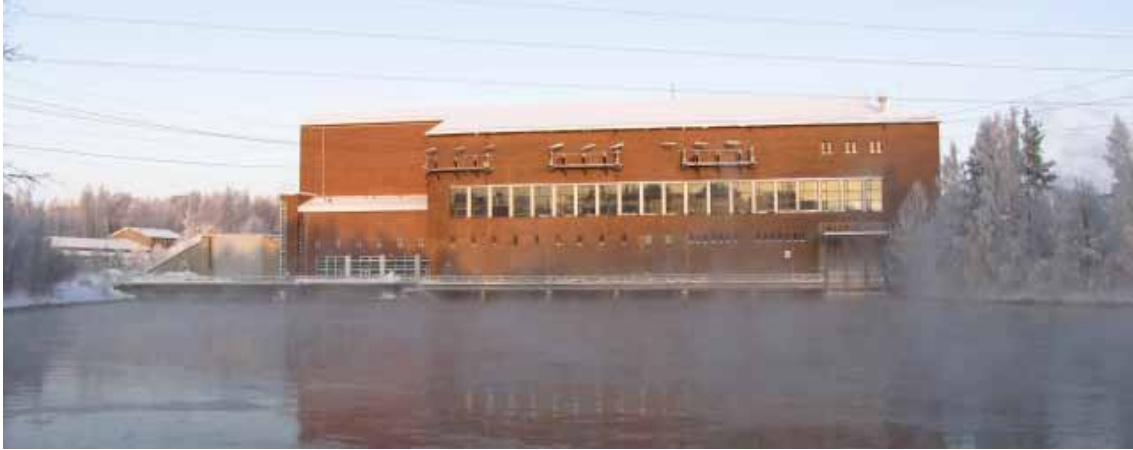
The Tainionkoski hydroelectric power plant in Imatra seen from downstream.
