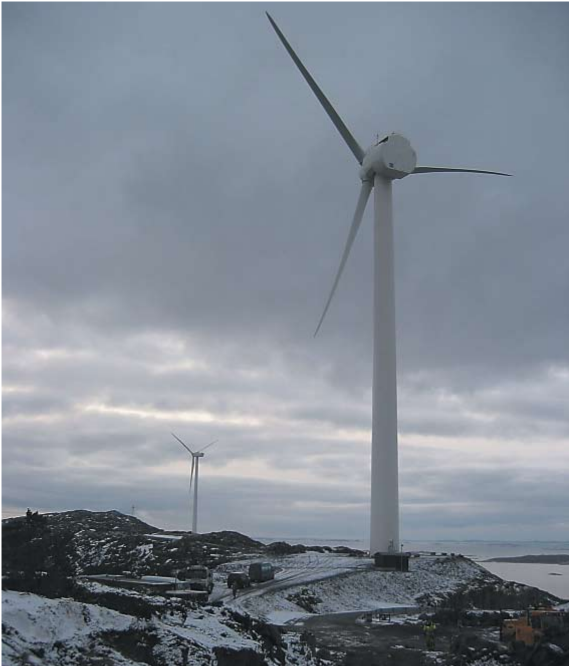
The Hundhammerfjellet wind farm is built to withstand the severe weather and wind conditions of the Norwegian west coast.
